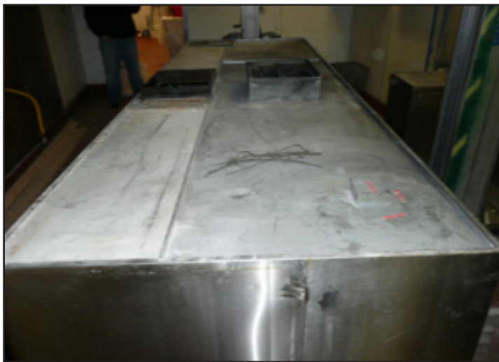
Grease hood removed and retrofitted so it could be reused.
